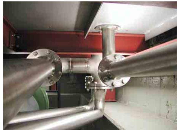
Under-floor piping: From the sockets in the floor of the dynamometer Bleyer has laid pipes to the emission measuring systems.
