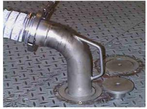
Adapter which connects the exhaust gas removal hose to the under-floor piping via the socket.
