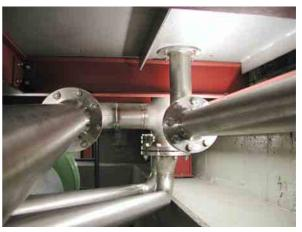
Under-floor piping: From the sockets in the floor of the dynamometer Bleyer has laid pipes to the emission measuring systems.
